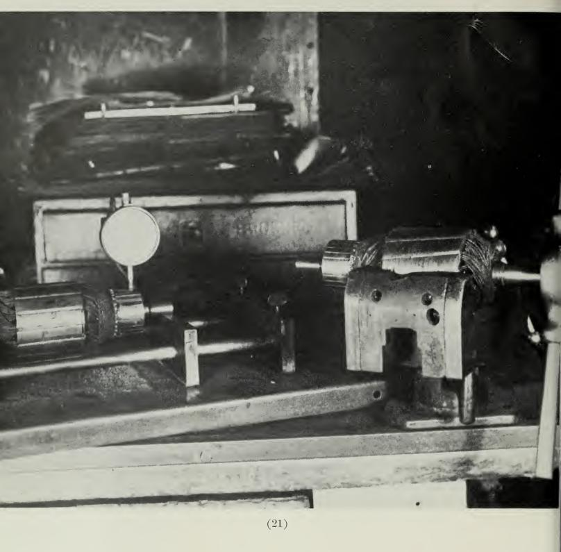
The armatures are then finally checked by rotating the commutators under a micrometer. This is done for the purpose of insuring that every bar of the commutator is of approximately the same height, otherwise proper contact with the generator brushes will not be made. This test is illustrated on the left side of the above picture.
